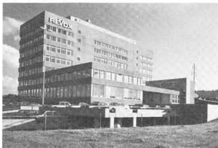
July 1976: move into the new production and administrative building
